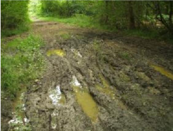
there is a section riddled with deep ruts and mud holes which were 4 to 5 metres wide and up to a metre deep. If you can imagine a large 360° digger getting stuck in the mud there, you get some idea of the extent of the damage making the route impassable.
